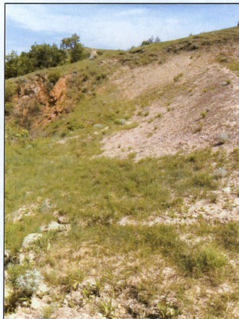
Photograph 6. Upper berm area (photo right) and lower berm (photo left). View to north.
